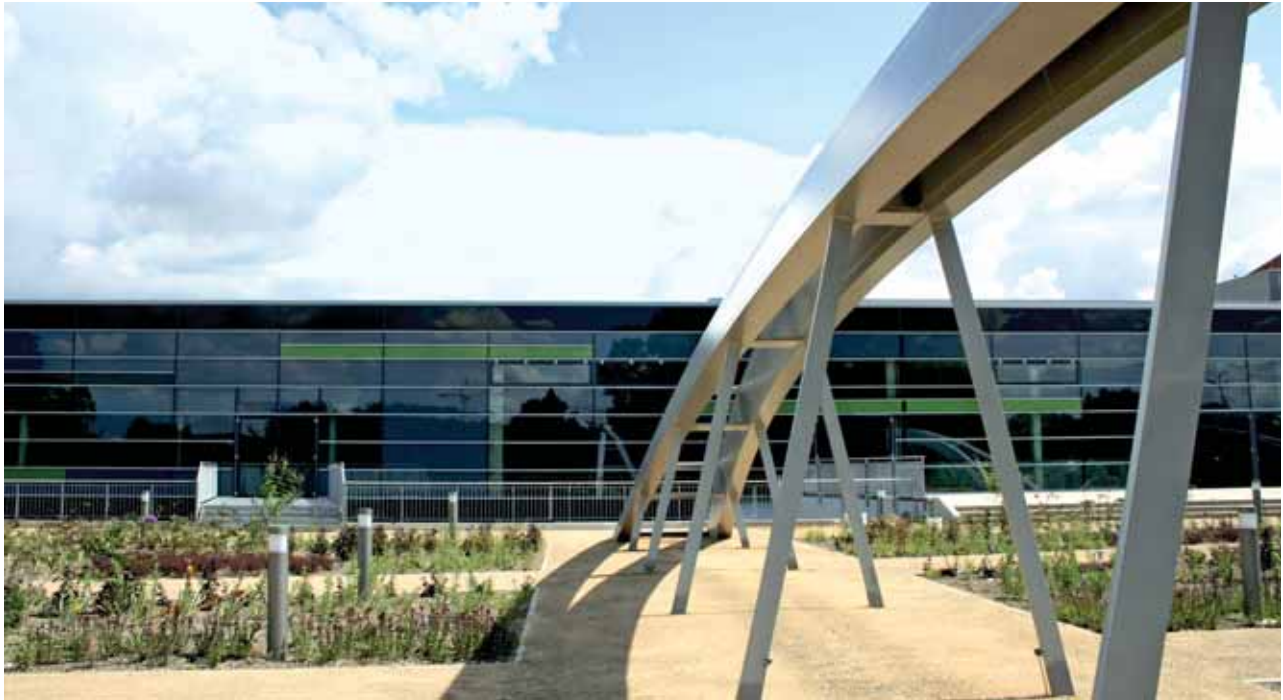
The multifunctional exhibition hall is spanned by reinforced concrete beams that are up to 46 metres wide
