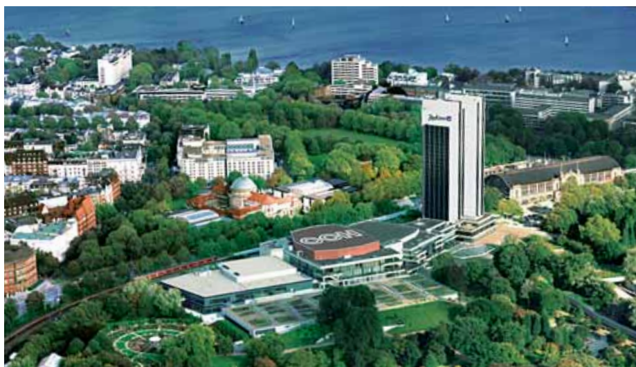
Europe's largest perennial rooftop garden has been planted on the roof of the CCH's multifunctional exhibition hall
