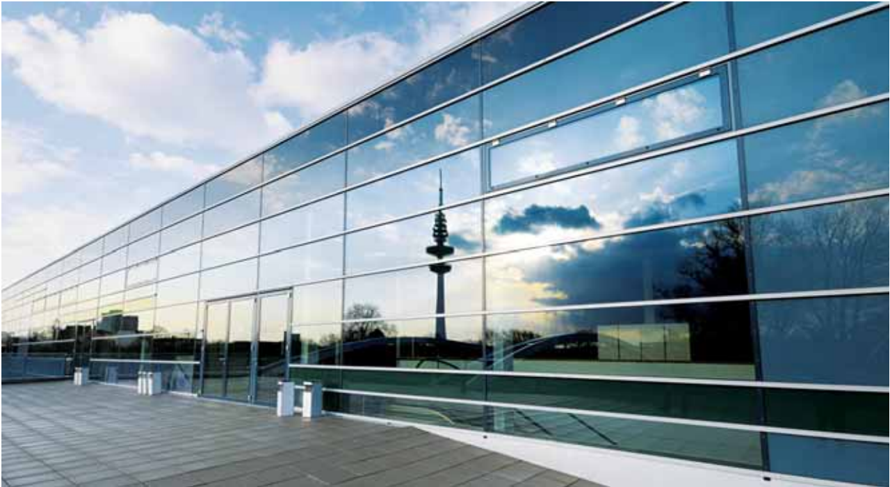
The new CCH possesses 10,000 square metres of exhibition space
