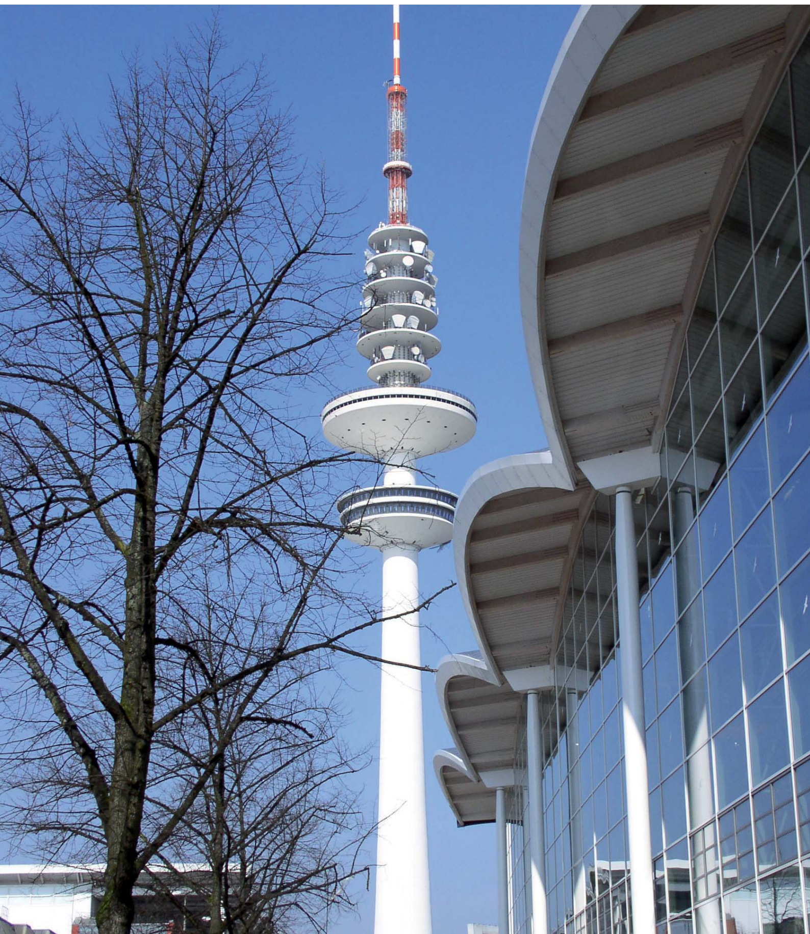
The new trade fair halls (r.) impress not only exhibitors. In combination with the TV tower, they are already one of the most popular photo motifs in Hamburg.
